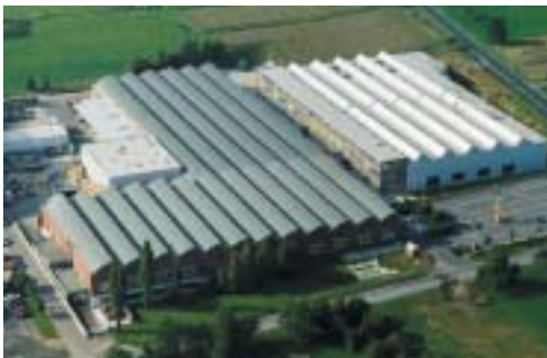
Niederahr, decanter production plant
